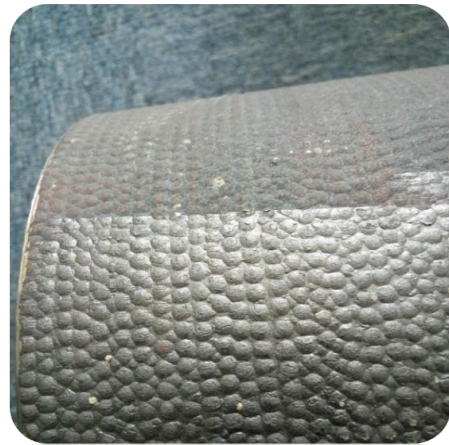
Steel member surface cleaning
